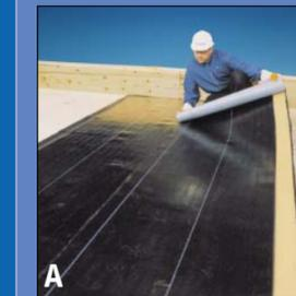
**A** Position the membrane before removing the release paper.
