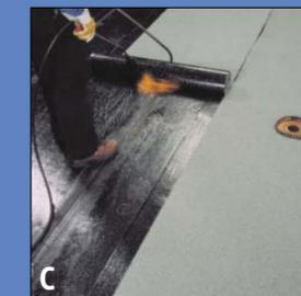
**C** Install cap sheet by heat welding or with Colply adhesive.
